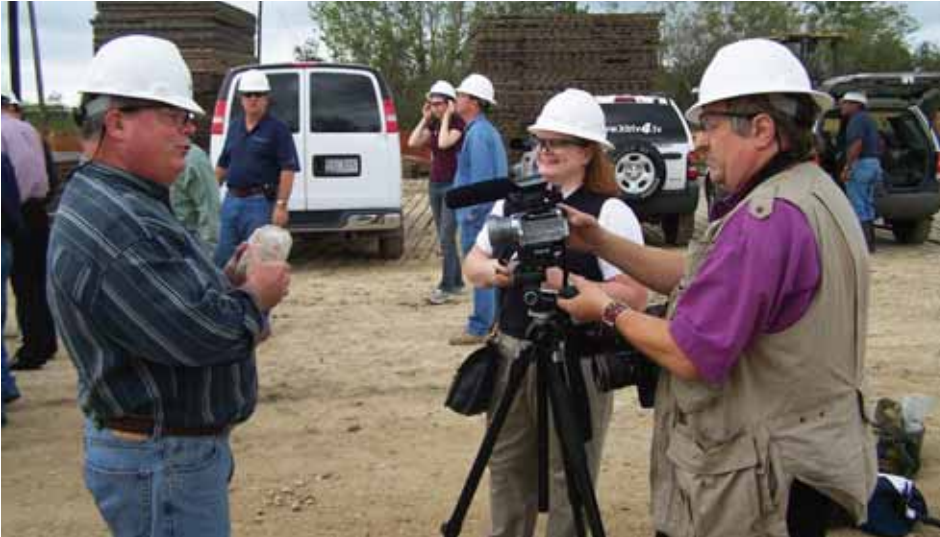
Golden Triangle Storage showed off its progress to local reporters and energy media from Houston Nov. 11. About a dozen reporters, photographers and videographers took advantage of the chance to see the construction process first hand, including climbing up to the three stories-high platform of the cavern drilling rig. AGL Resources' David Schultz displays a salt core from Spindletop to Houston Chronicle reporters.
